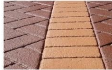
COLORLED AND STAMPED ASPHALT CROSSWALK
